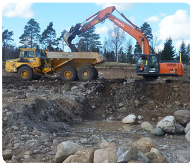
Schaktning i Grimstorp (Foto: Roger Siverth)
